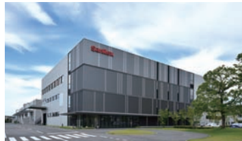
● Shiga Plant (Power supplies)
